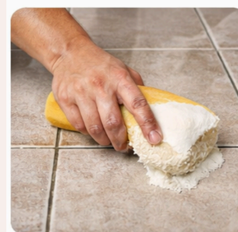
Final cleaning and wiping of tiles for a neat finish.
