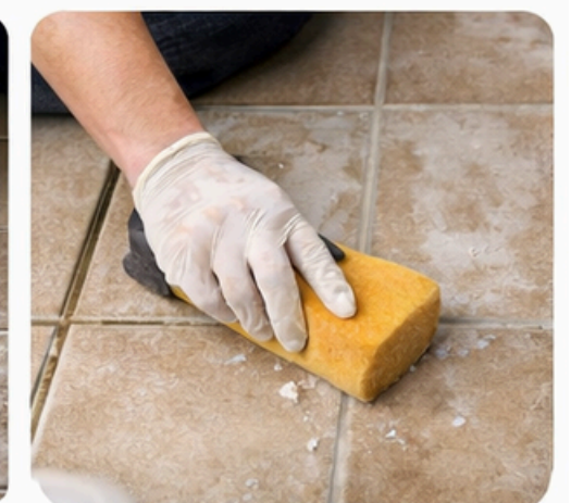
Removing excess grout from tile surface with a damp sponge.
