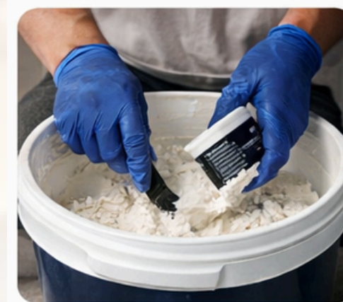
Mixing the epoxy grout thoroughly using a spatula until a smooth, uniform paste is formed.
